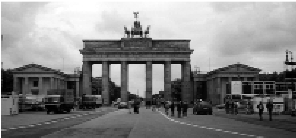
Brandenburg Gate, which once divided East and West Germany
